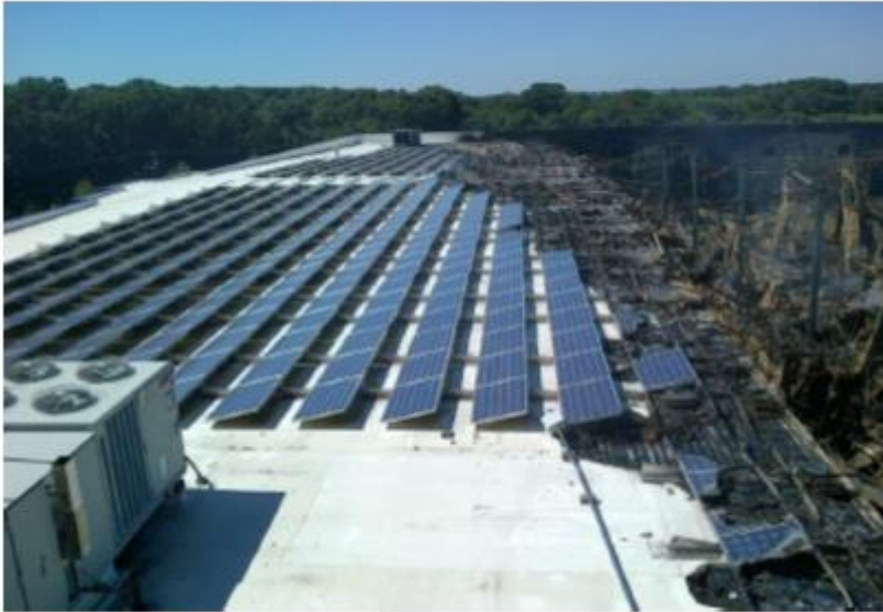
Aftermath of Delanco, NJ, Warehouse Fire. Source: New Jersey State Fire Marshal, 2013
